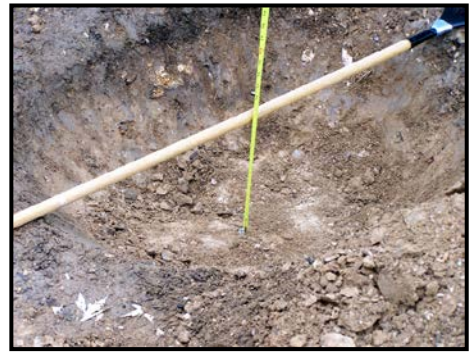
Figure 7. In digging, measure the depth of the planting hole with a straight board (like rake handle) and a measuring tape.
